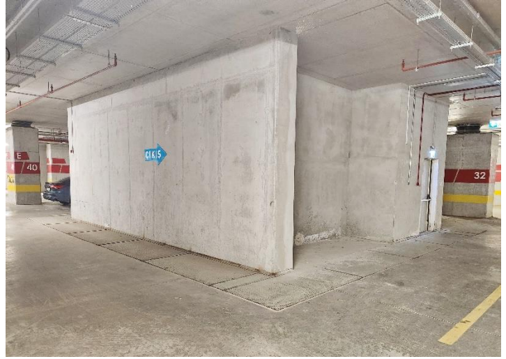
Seismic joint cover around elevator/stairway shaft in basement
