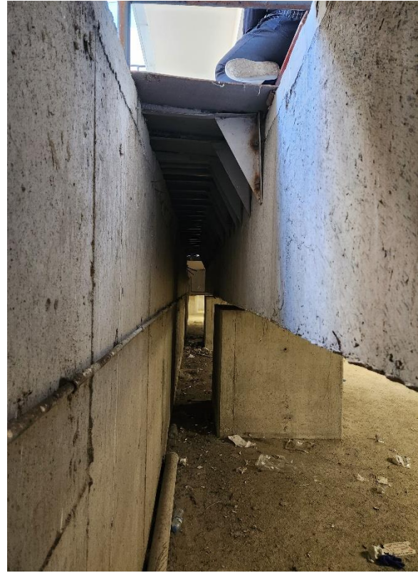
Perimeter joint and moat cover, view from under side
