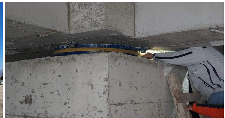
Inspection of isolation bearing using boroscope
