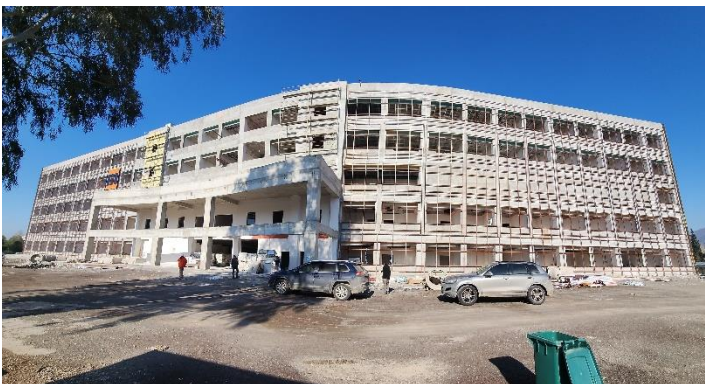
Status of construction at time of earthquake
