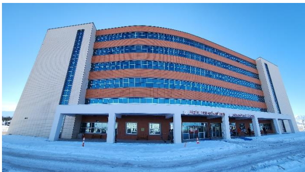
General view of hospital at time of post-earthquake inspection visit
