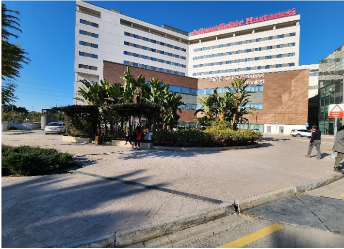
General view of hospital and seismic joint in foreground
