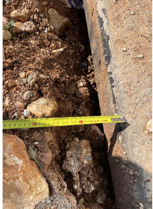
Estimated maximum displacement approximately 12 cm
