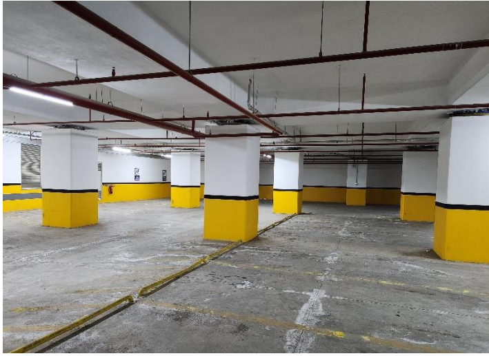
General view of isolation basement
