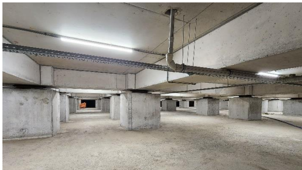
General view of isolation basement
