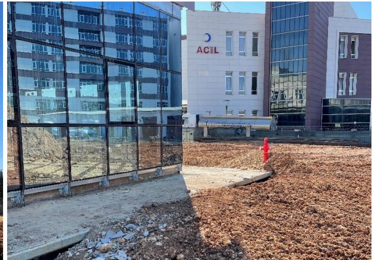
Soil fill at moat cover perimeter
