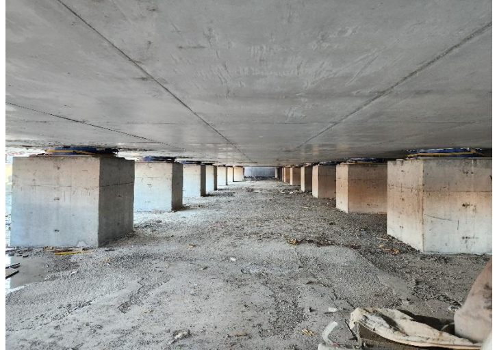
General view of isolation basement
