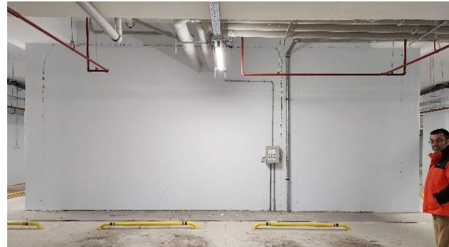
General view of isolation basement
