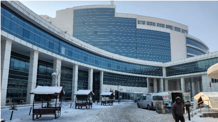
General view of hospital at time of post-earthquake inspection
