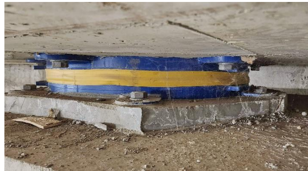
Double pendulum bearing, with small residual offset visible
