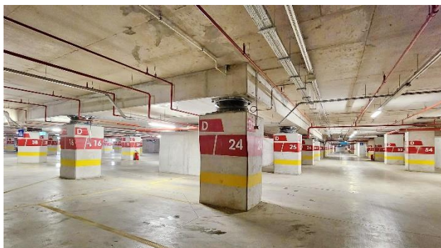
General view of isolation basement
