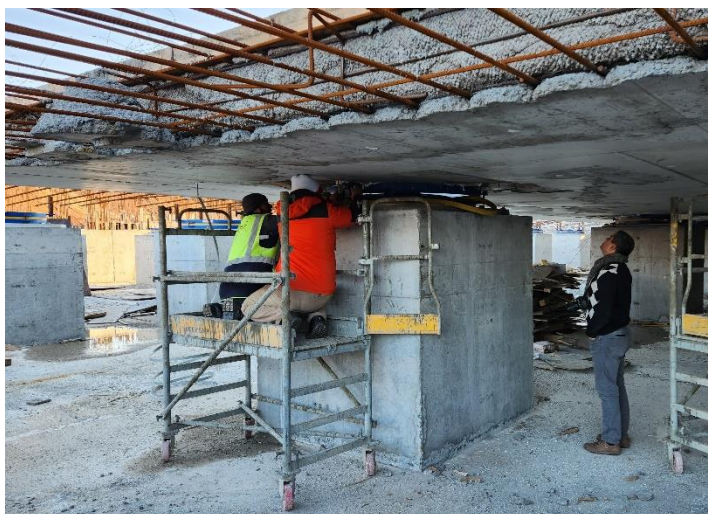
Inspection of isolation bearing with boroscope
