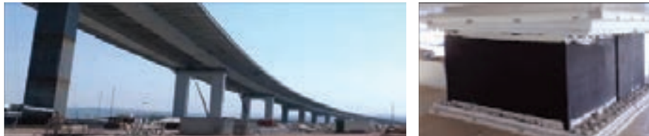
Figure 16. General view of South Approach Viaduct and the LRB units used
