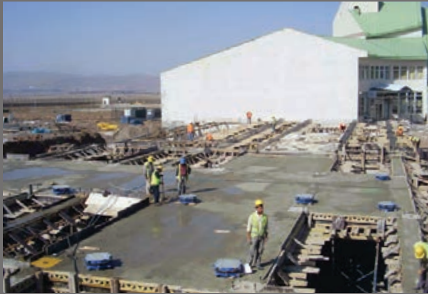
Installation of isolators at the main block
