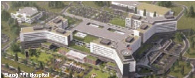
Elazığ PPP Hospital
