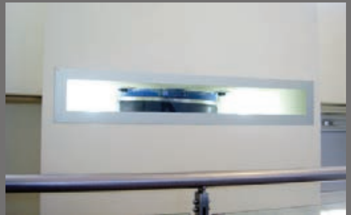
Some isolators were surrounded by glass frame for display purposes
