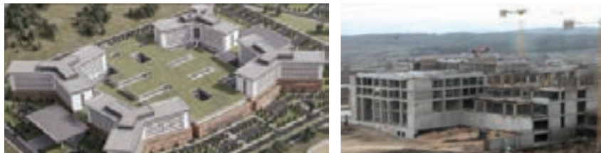
Figure 11. Bursa City Hospital
