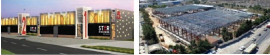
Figure 14. Star of Bosphorus Data Center
