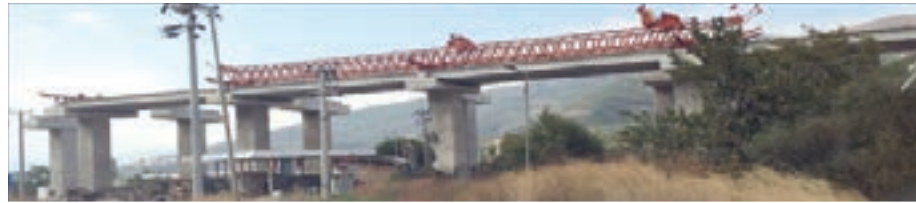
Figure 18. General view of Gemlik Viaduct of the Gebze-İzmir Highway
