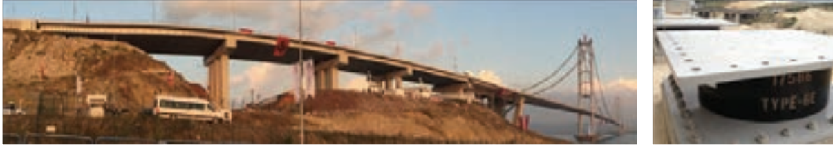
Figure 17. General view of South Approach Viaduct and the LRB units used
